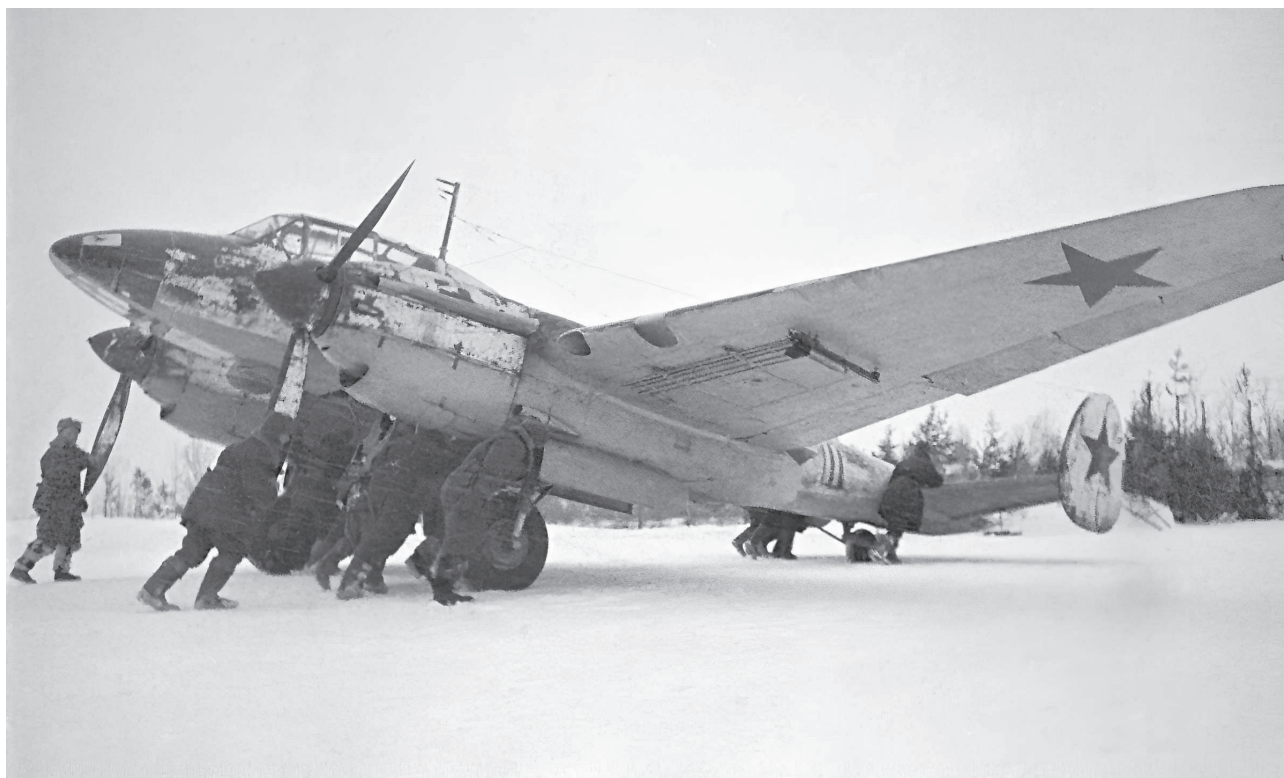
A Soviet Pe-2 bomber after a combat mission. Note the dive brakes under the wing and the open bomb bays.
